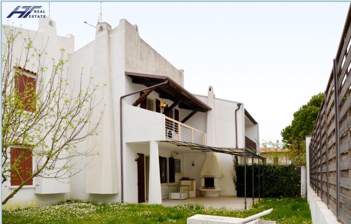
back facade from private garden
