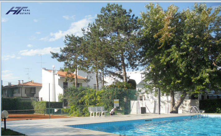
residential units from swimming pool
